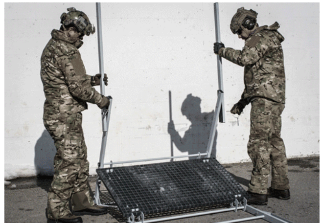
Figure 4 - Rotate uprights
