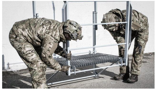
Figure 9 - Secure railing bolt
